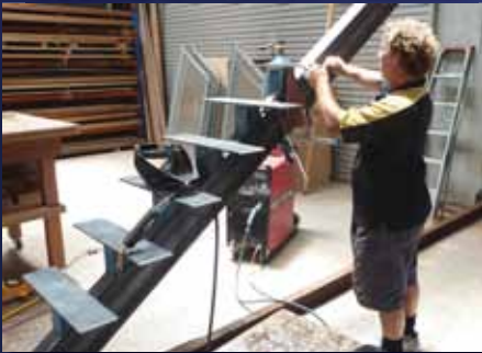
Setting out stairs ready for welding
