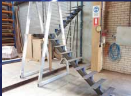
A fully welded system ready to be disassembled
