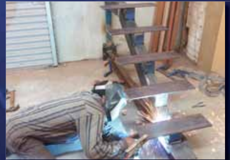
Heavy duty mig welding.
