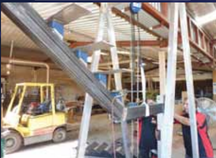
Stairs being positioned and lifted with block & table
